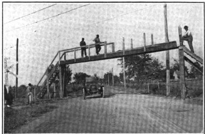
One of the numerous small bridges adding to safety of the course
